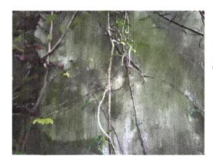
**Inspection:** Internal wall showing overgrown vegetation is causing the walls to crack.
